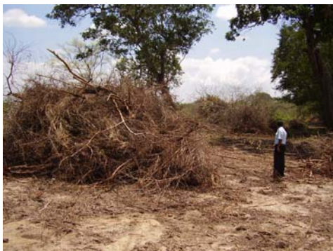
Uprooting and removing of Prosopis by using machinery
